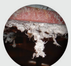
Spray-on Insulation
