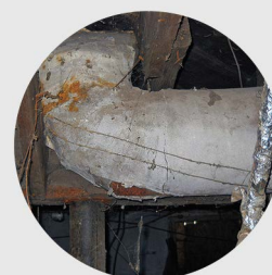
Heating System Insulation
